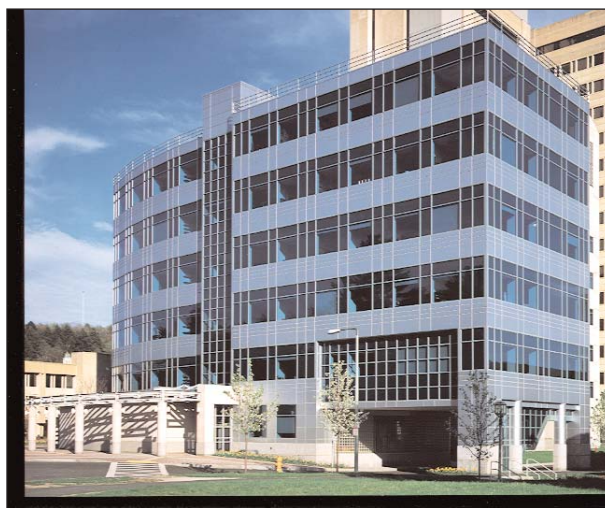
Silvio O. Conte National Center for Polymer Research on the UMass/Amherst campus. The office wing (above - 39,000 sq.ft.) is connected to a laboratory complex (133,000 sq.ft.) and houses the complete Polymer Science & Engineering Department, the Materials Research Science & Engineering Center (MRSEC), and the Center for the University of Massachusetts Industry Research on Polymers (CUMIRP).
